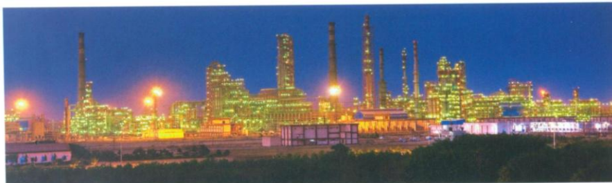
Essar's Vadinar Refinery
